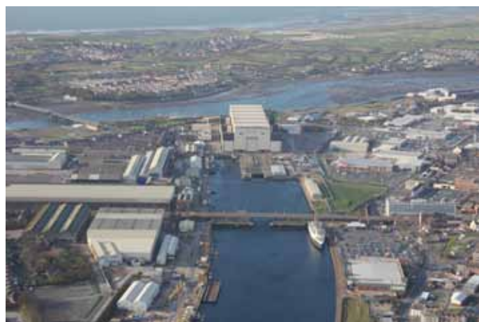
Naval shipbuilding facility - Devonshire Dock Hall, Barrow in Furness (photo courtesy of Furness Enterprises)
